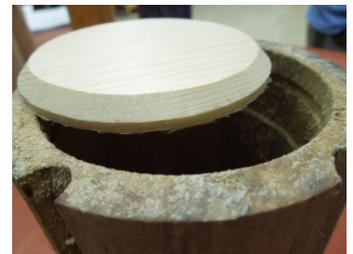
The photo above on left, show the internal groove that accepts the "snap fit" of the box bottom. The photo at right shows the box bottom before snapping it into the body groove. The angle and clearances between the bottom and internal groove are based on experience factored on wood age, condition, size, etc., to arrive at a snug fit when dried.
